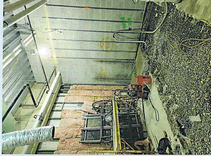
Classroom/New bathroom area: Removal of 8" thick concrete floor and saw cutting the new doorways
