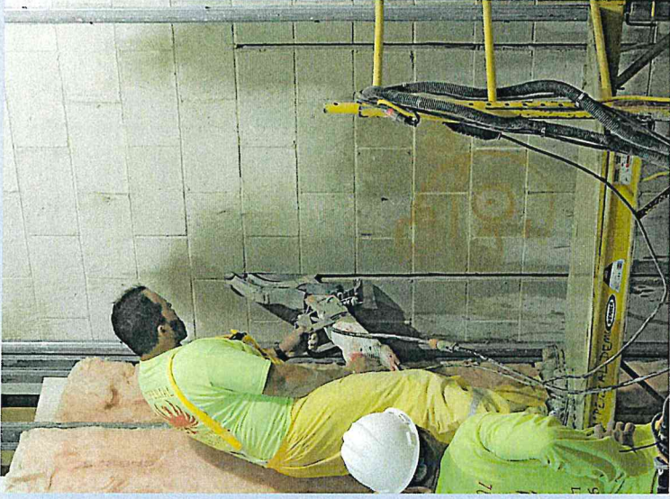
Continuation of saw cutting and the removal of the block wall for the new doorways
