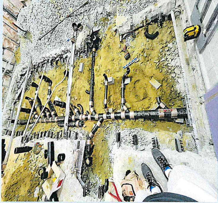
Rough plumbing for waste drains for the new bathrooms
