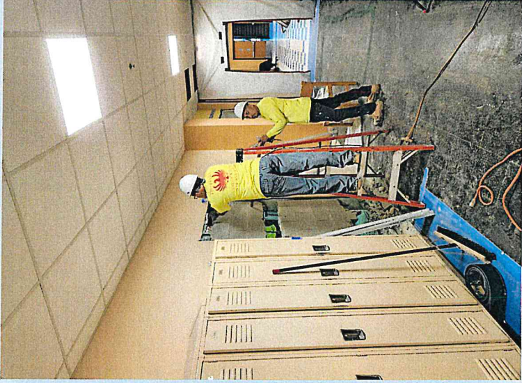
Continuation of saw cutting and the removal of the block wall for the new doorways
