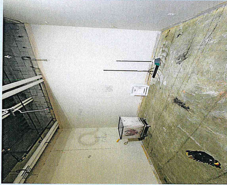
Classroom area: the removal of the flooring, ceiling, and saw cutting the floor for the new plumbing
