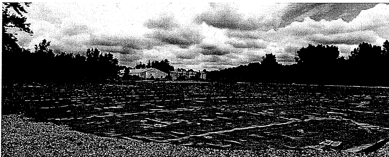
View looking north towards the former manufacturing areas of the Olin Chemical Superfund Site. Visible in the foreground is the temporary cap on the Slurry Wall Containment Area.
