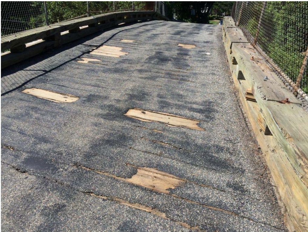
Photo 2: Typical wearing surface, exposed deck planks.
