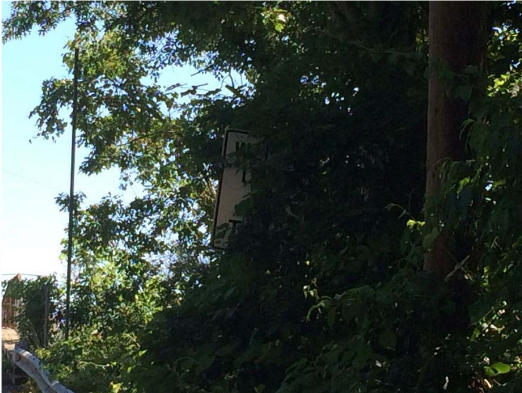
Photo 1: West elevation, hidden "At Bridge" Weight Posting Sign.
