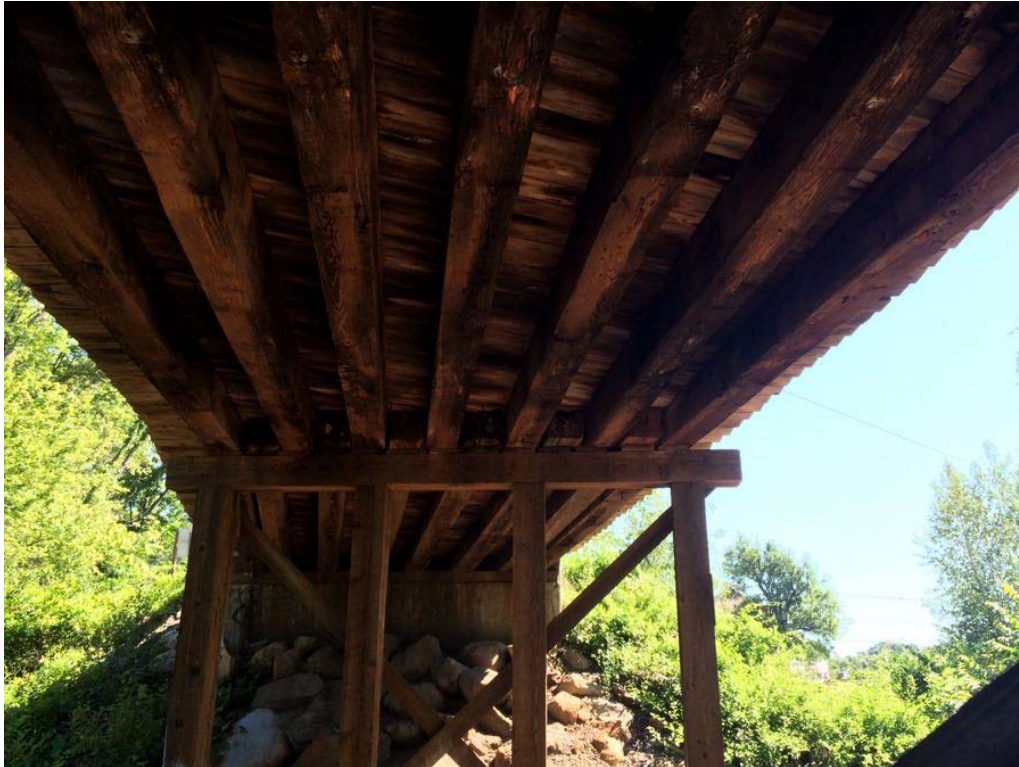
Photo 11: Span 2, typical underside.
