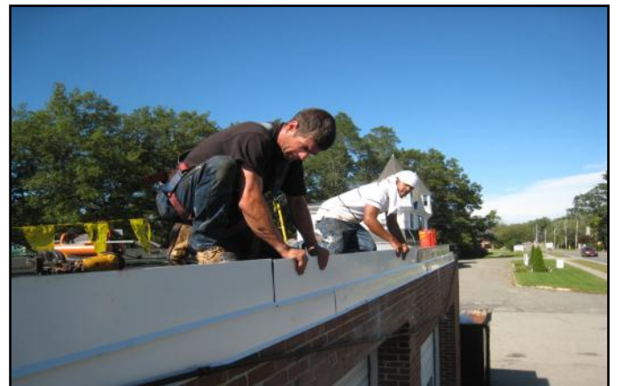
Above: Walls were flashed with an elastomeric reinforced flashing sheet.
