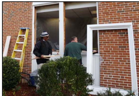
Wilmington Memorial Library window and door replacement project
