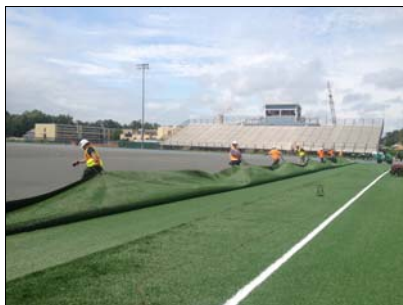
Construction of Artificial Turf Field
