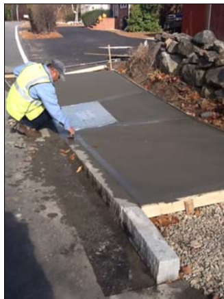
Installation of ramp on Woburn Street Sidewalk
