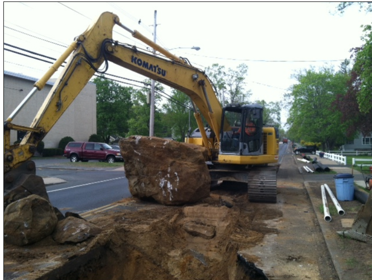
Sewer Main Installed for Connection to the New High School
