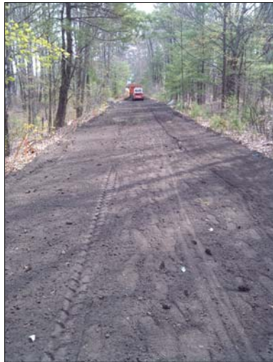
Restoration of Degraded Floodplain Wildwood Street Pedway
