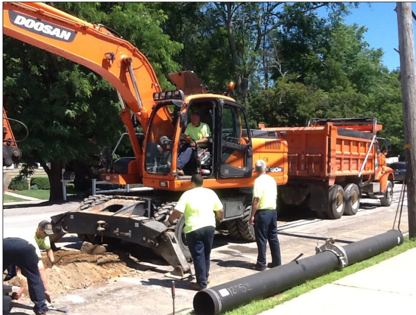
Church Street water main upgrade
