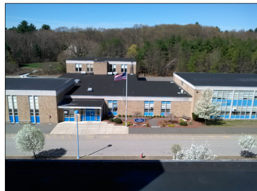
New roof was installed at the West Intermediate School
