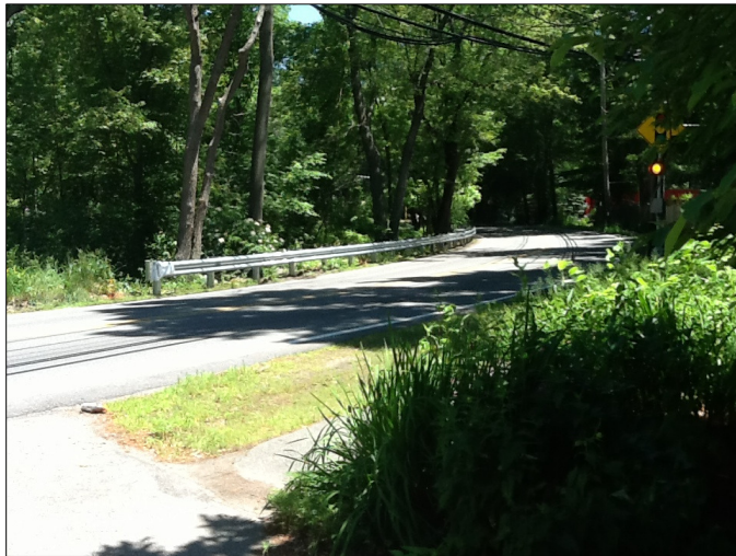
New guardrail installed on Burlington Avenue with use of WRRRP funding
