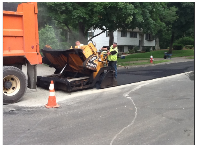
Roadway repairs on Lucaya Circle
