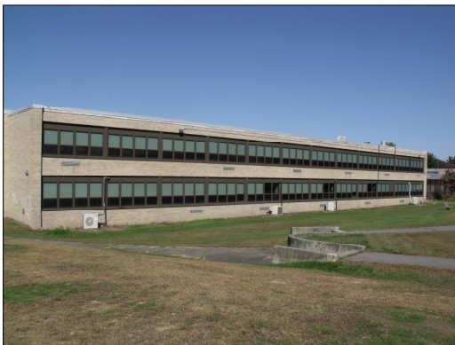
New windows were installed at the North Intermediate School
