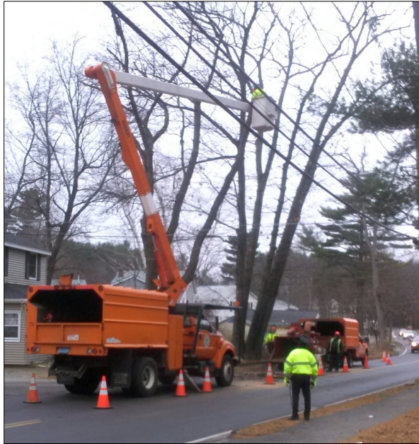
Tree Division employees performing maintenance work on Glen Road
