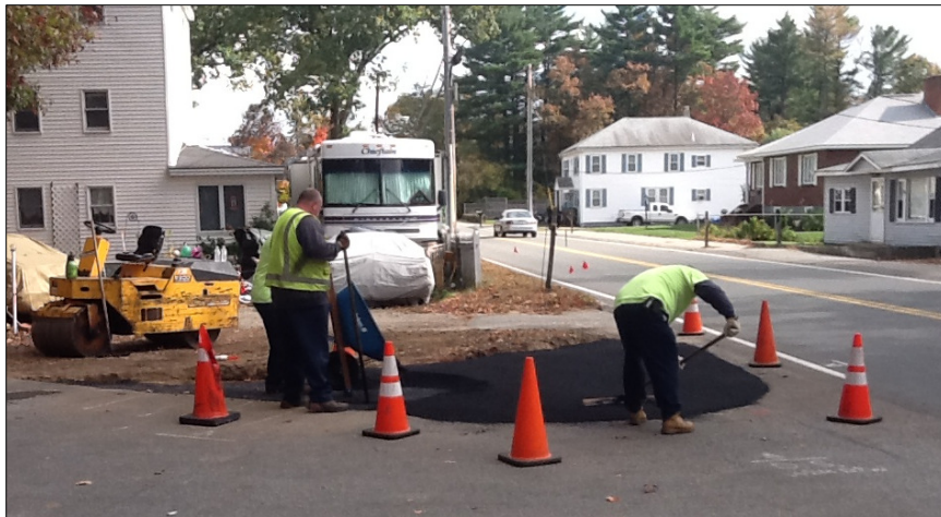
DPW employees construct wider turning radius at Oak Street
