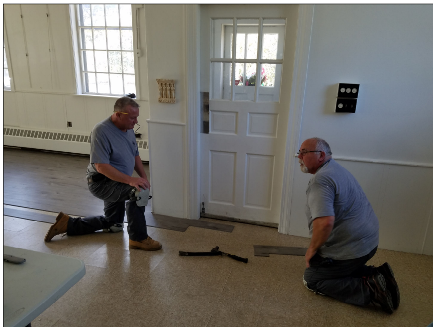
Gordon Fitch and Barry Ferrara install new flooring at Arts Center
