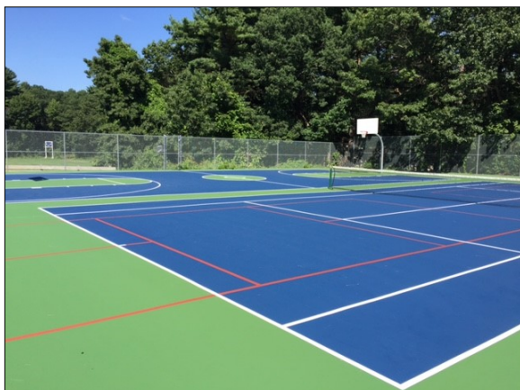
Newly Resurfaced Court Lined for Pickleball.
