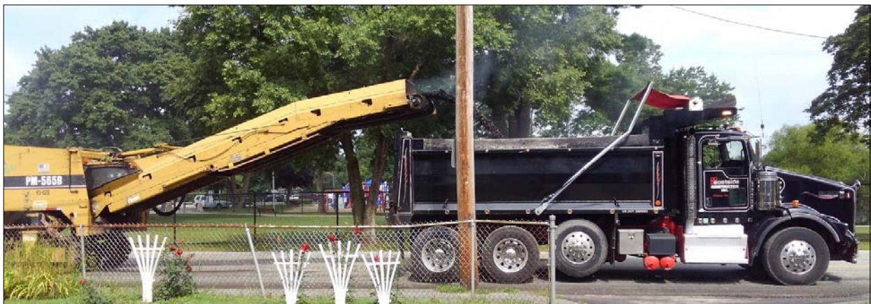
Resurfacing of Grove Avenue.
