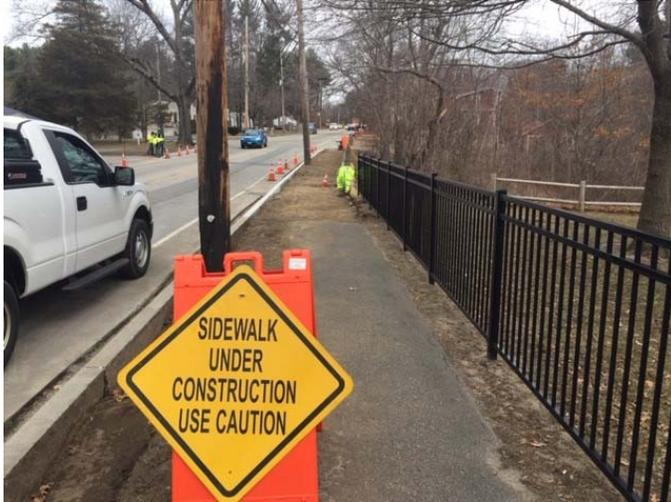
New granite curbing was installed on Middlesex Avenue between Glen Road and Colonial Drive, with portion of existing granite curbing getting reset to proper height. This work started March 27, 2019 and finished April 1, 2019. D&R Contracting, the Town's FY 19 Roadway Management Contractor, performed the work. Approximately 650 linear feet of new granite curb was installed, and 450 linear feet of existing granite curb was reset.
